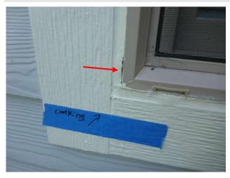
Close-up photo of condition shown previously illustrating sealant void (left), and missing railing end caps (below).
