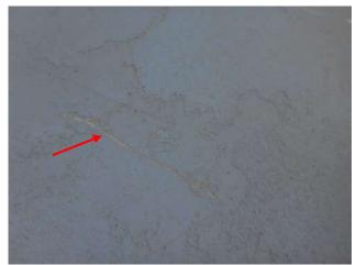
Additional photo of condition shown previously illustrating damage to deck coating.
